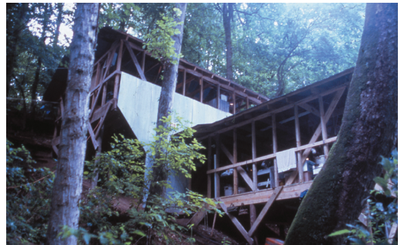
FIGURE D6.10 The kitchen (upper) and laboratory (lower) facilities that were constructed at the Dust Cave field camp.
