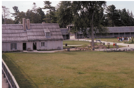
FIGURE D8.2 Excavations of House D in progress at Fort Michilimackinac, with reconstructed Houses AB and C on the left.
